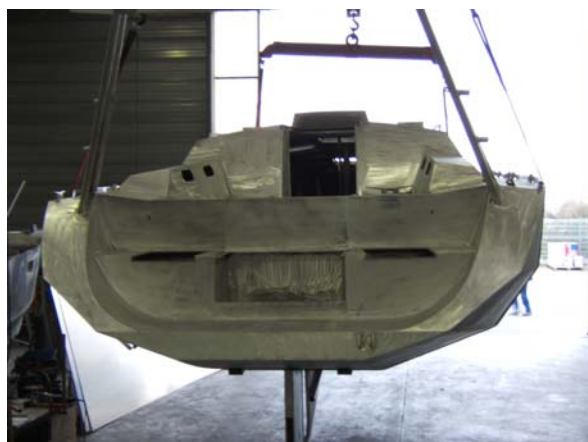
An Ovni 365 at the end of welding
